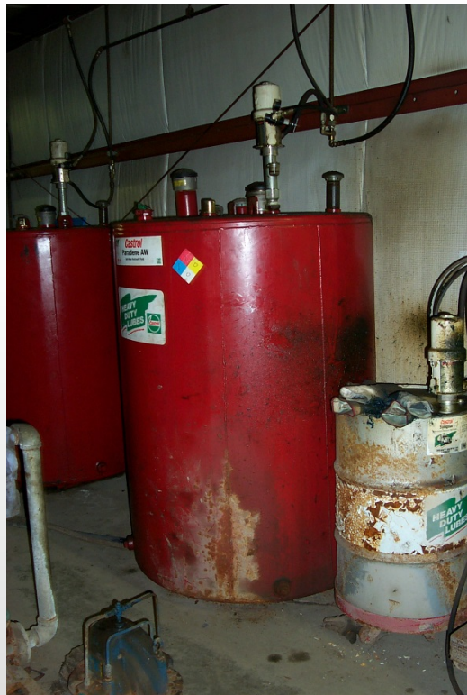
Bulk oil tank and oil transfer
